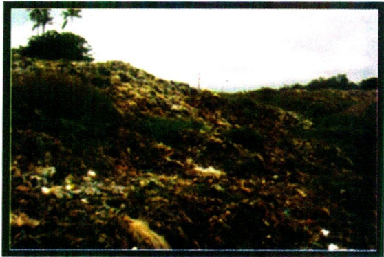
Fig 3. Gohagoda open dumping site
